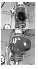
4) Replace the gasket/O-ring of the housing.
