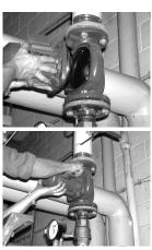
3) Lift the operation unit from the pump housing. Watch out for hot water!
